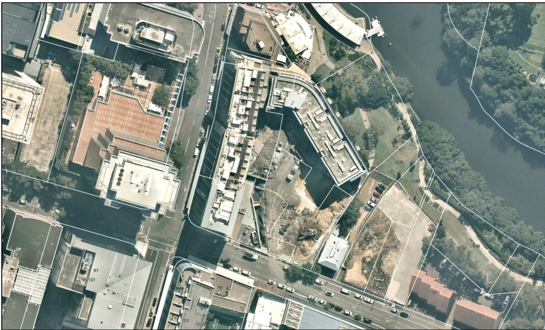
Figure 3: Aerial view of the site (NearMap 7 April 2019). Block A has been demolished in this image.
